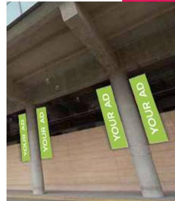
Banner – Infield Tram Column
